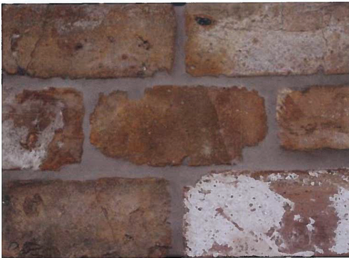
Cracked & Chipped Bricks – After Installation
