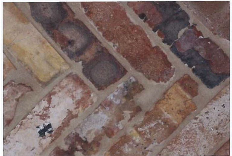
Cracked & Chipped Bricks – After Installation
