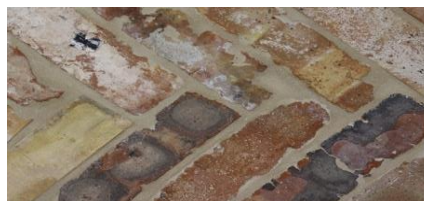
Cracked & Chipped Bricks – After Installation
